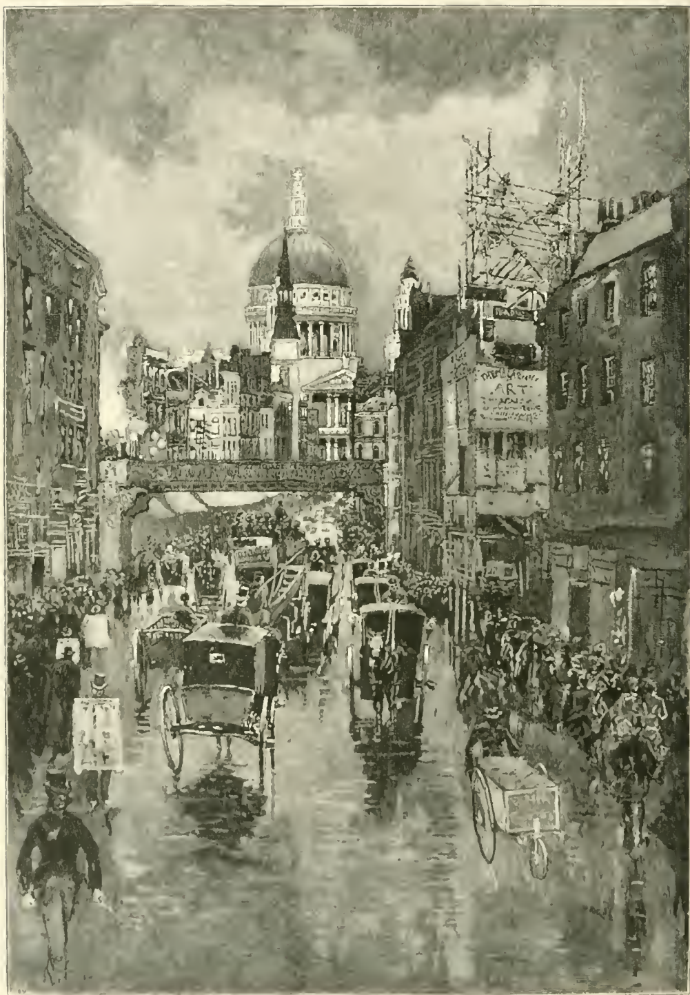
THE WEST FRONT OF ST. PAUL'S, FROM LEFT STREET.
